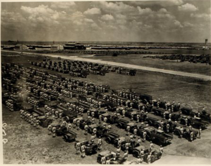
Standing by for inspection.
