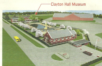
South end view.
